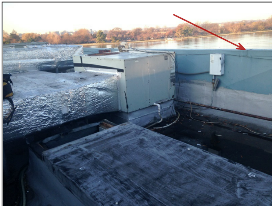
4 - View of Asbestos-Containing Black Parapet Coping Sealant on the Roof of the Pier 3 Office Building. Sample No. R5.
