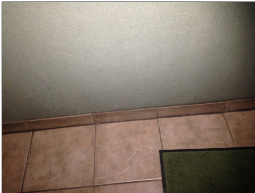
6 - View of Lead-Based Glaze on Tan Ceramic Floor Tile and Baseboard in the Bathroom. XRF Reading 26 and 43.
