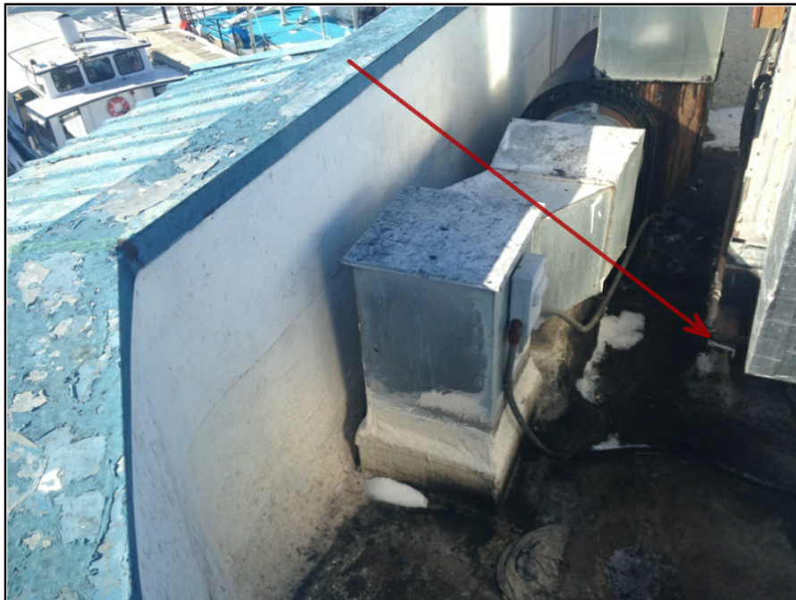
6 - View of Asbestos-Containing Roof Pitch Pocket on the Roof of the Cantina Marina Building. Sample No. R11.
