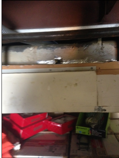
3 - View of Asbestos-Containing White Mastic associated with Silver HVAC Insulation Wrap in the 1st Floor North Electrical Room of the Pier 3 Office Building. Sample No. 7.
