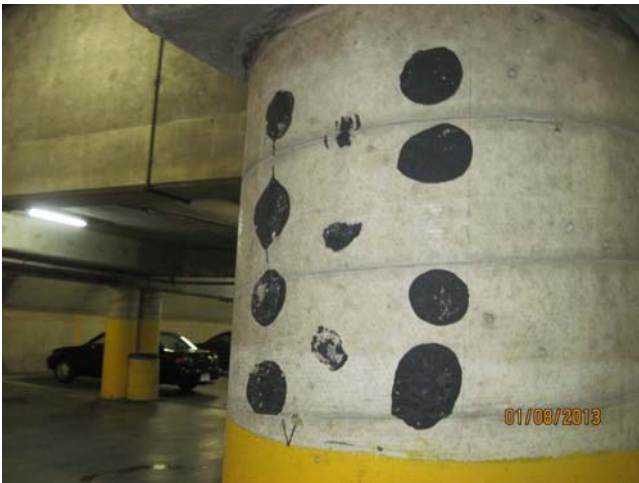
9. View of black glue dots on concrete columns within the garage. Samples CI84-CI86
