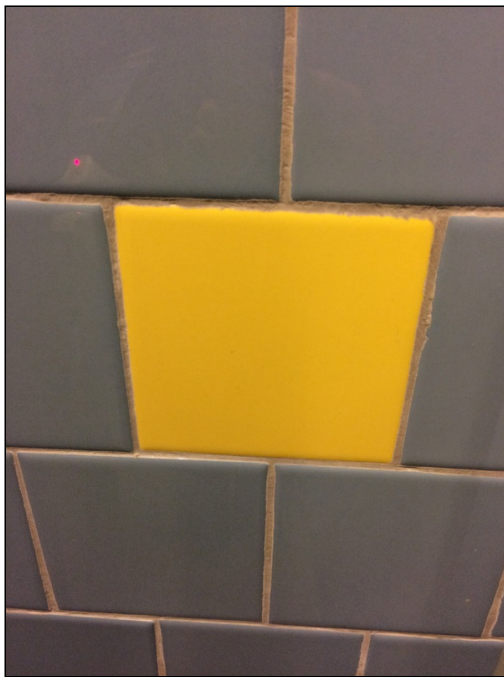
10 - View of Lead-Based Glaze on Yellow Ceramic Wall Tiles in the Restroom of Cantina Marina. XRF Reading No. 52.
