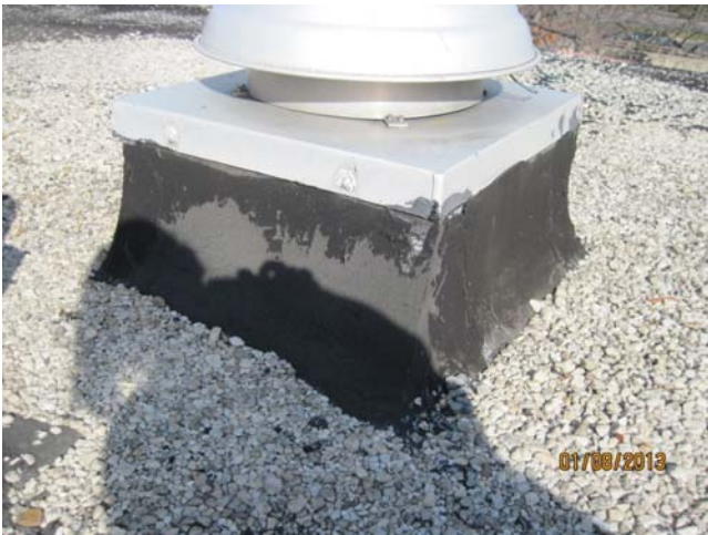
3. View of the black tar over the roof hood flashing on the lower roof. Samples CI53-CI55
