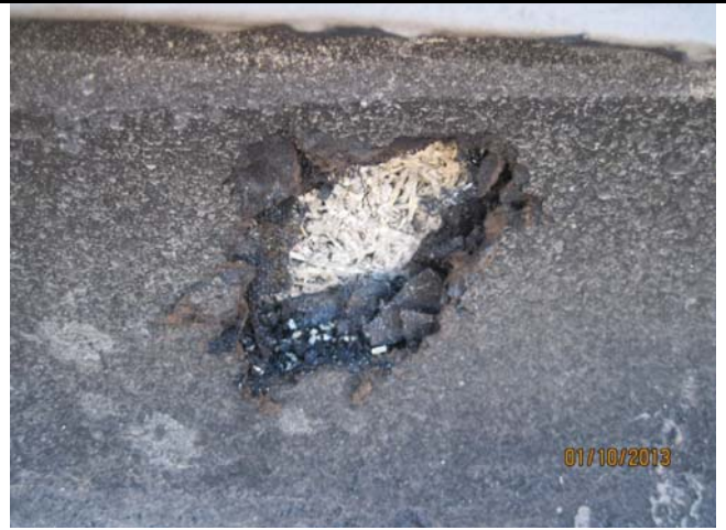
8. View of the lower roof flashing, the first and second layers are positive. Samples CI101-CI107
