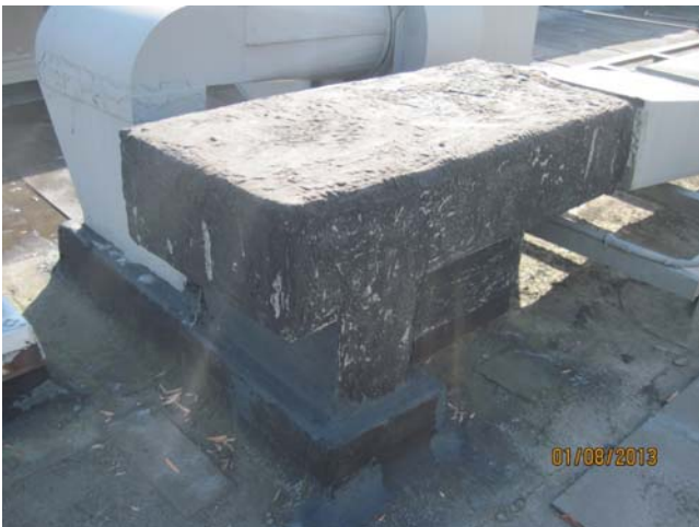
5. View of the black tar over mechanical hood. Samples CI69-CI71
