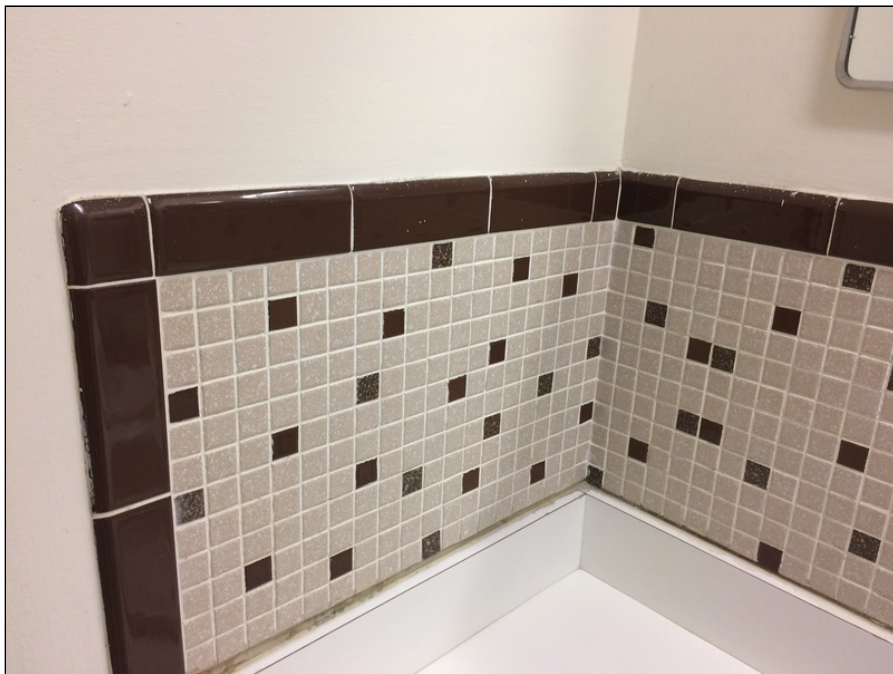
8 - View of Lead-Based Glaze on Brown Ceramic Wall Tiles in the 2nd Floor Restroom of the Pier 3 Office Building. XRF Reading No. 18.
