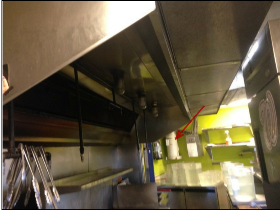
15 - View of Fire Suppression System in the Kitchen of Cantina Marina.
