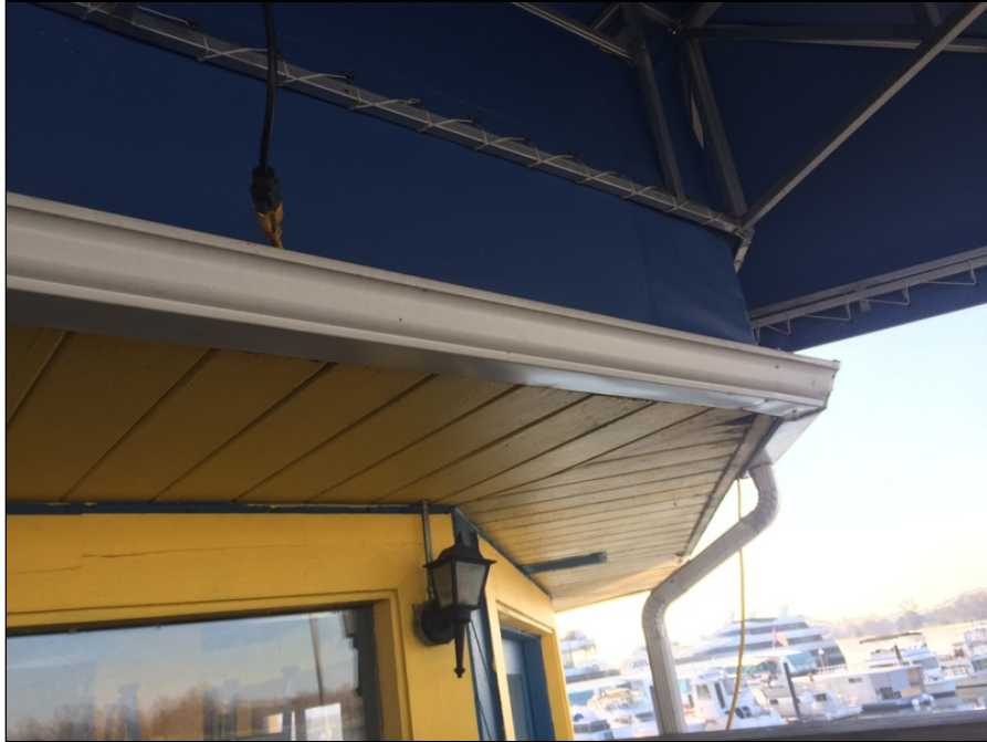
13 - View of Lead-Based Paint on White Metal Crown Molding in the 2nd Floor of Cantina Marina. XRF Reading No. 69.
