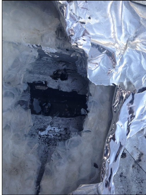
5 - View of Asbestos-Containing Gray/Black HVAC Sealant beneath Foil/Plastic Insulation on the Roof of the Pier 3 Office Building. Sample No. R9.
