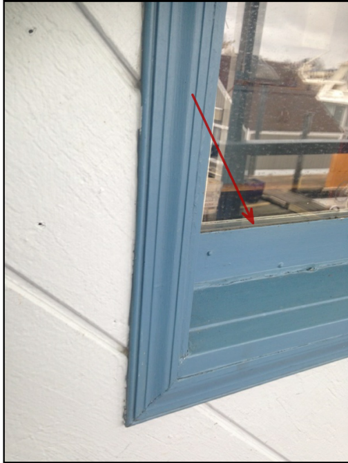
5 - View of Asbestos-Containing Exterior Gray Window Glaze on the West Exterior of the Building. Sample No. 13.
