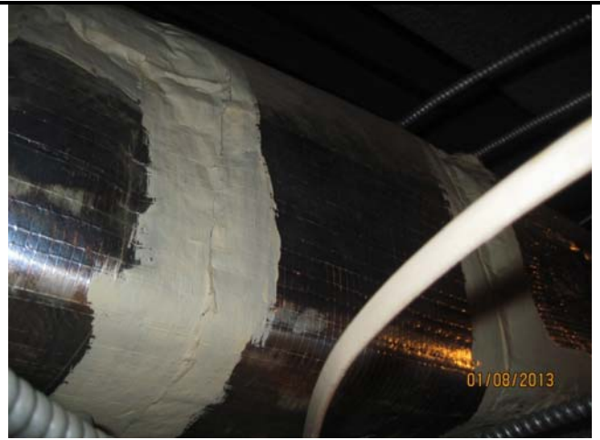
2. View of the white duct seam mastic above drop ceilings throughout the building. Samples CI42-CI44
