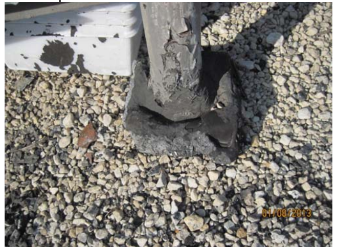
4. View of the black pitch pocket material on the lower roof. Samples CI56-CI58
