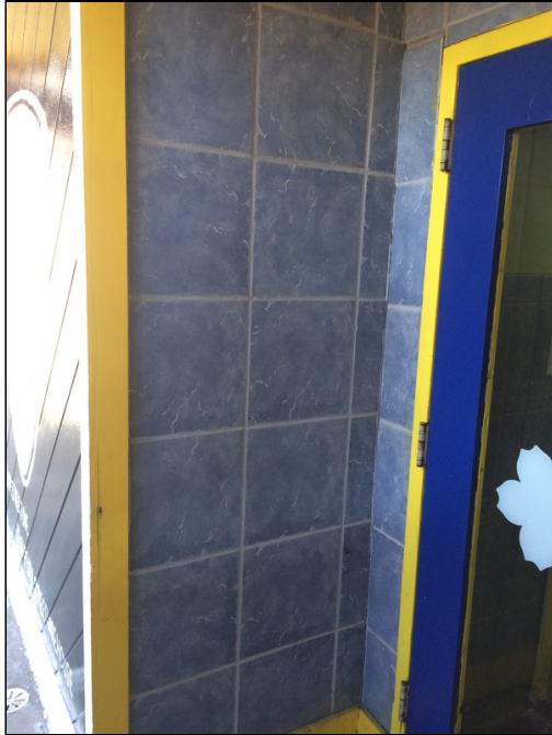
9 - View of Lead-Based Glaze on Blue Ceramic Wall Tiles in the Exterior Bar Area of Cantina Marina. XRF Reading No. 44.
