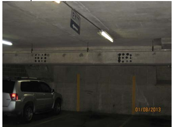
10. View of black glue dots on concrete supports within the garage. Samples CI84-CI86
