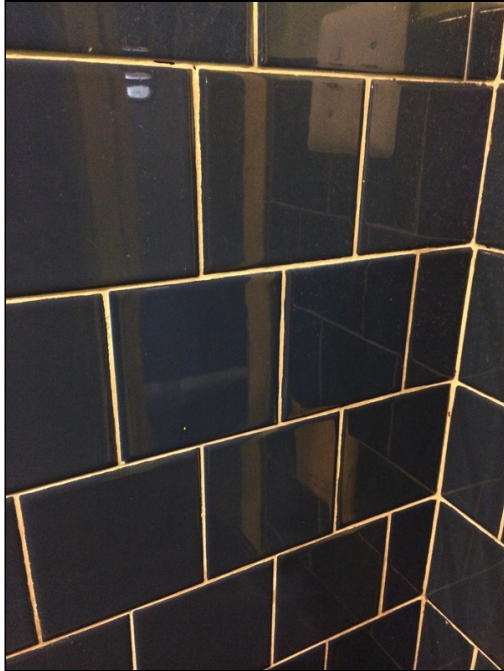
11 - View of Lead-Based Glaze on Blue Ceramic Wall Tiles in the Restroom of Cantina Marina. XRF Reading No. 55.
