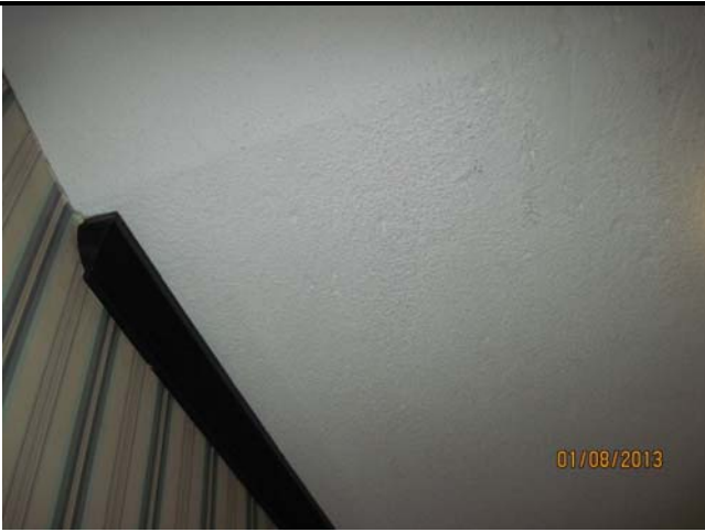
1. View of the textured ceiling plaster within the lobby hallway. Samples CI31-CI35
