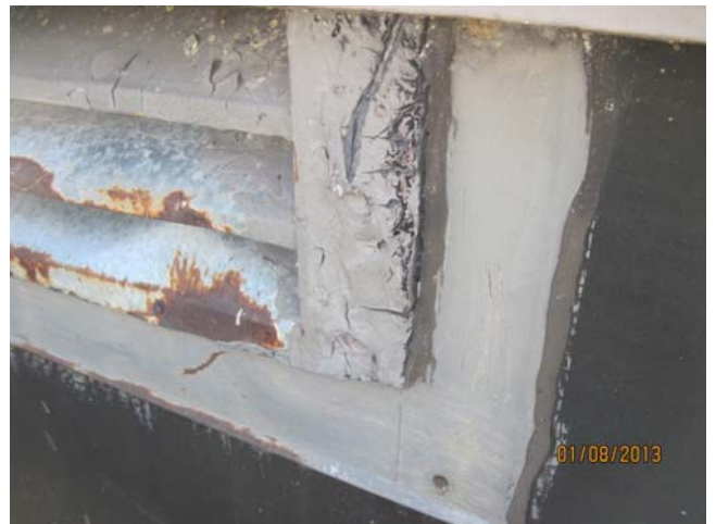
6. View of the black caulk around roof air vent. Samples CI75-CI77
