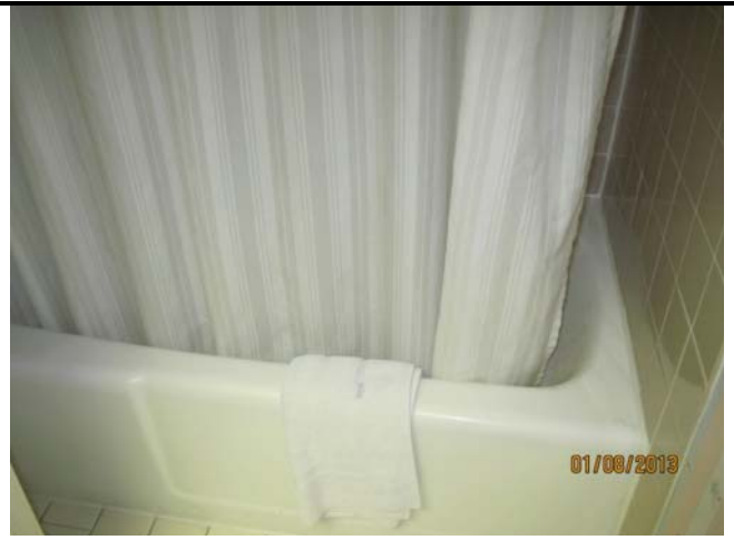
14. View of the beige/white lead coated ceramic tubs.
