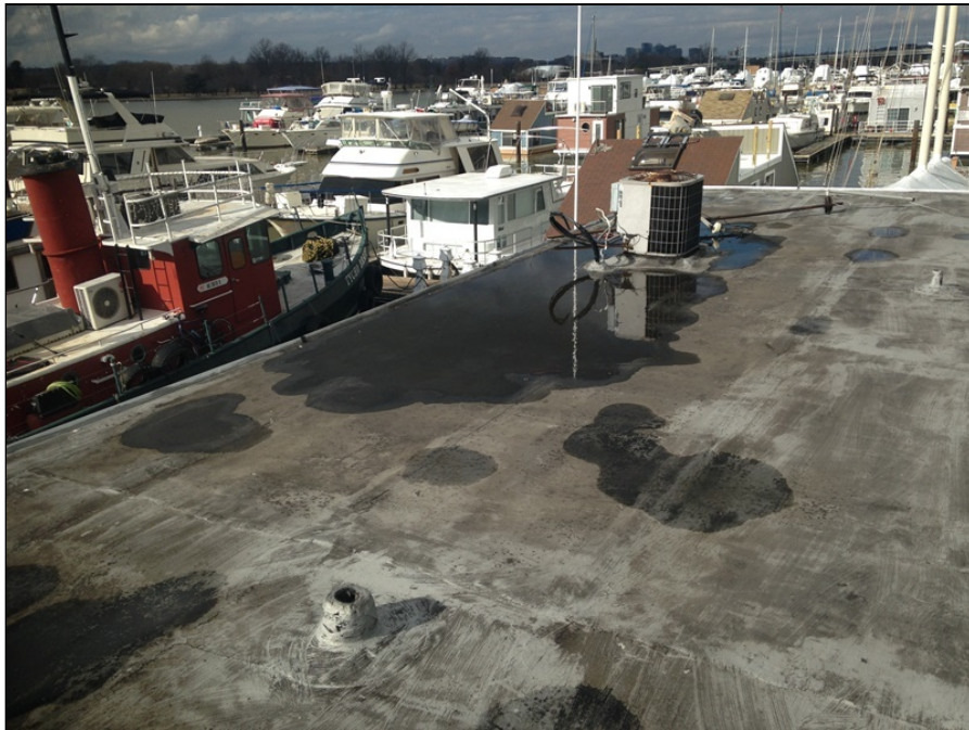
4 - View of the Roof of the Building.
