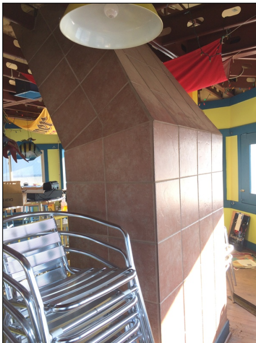
12 - View of Lead-Based Glaze on Pink Ceramic Wall Tiles in the 2nd Floor of Cantina Marina. XRF Reading No. 62.
