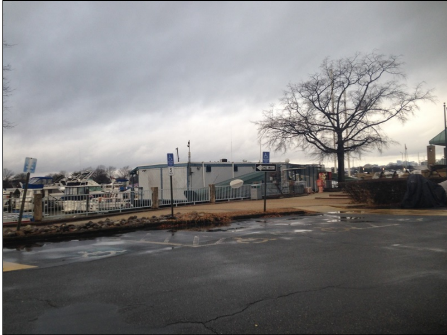
1 - View of Pier 3 Security Building.
