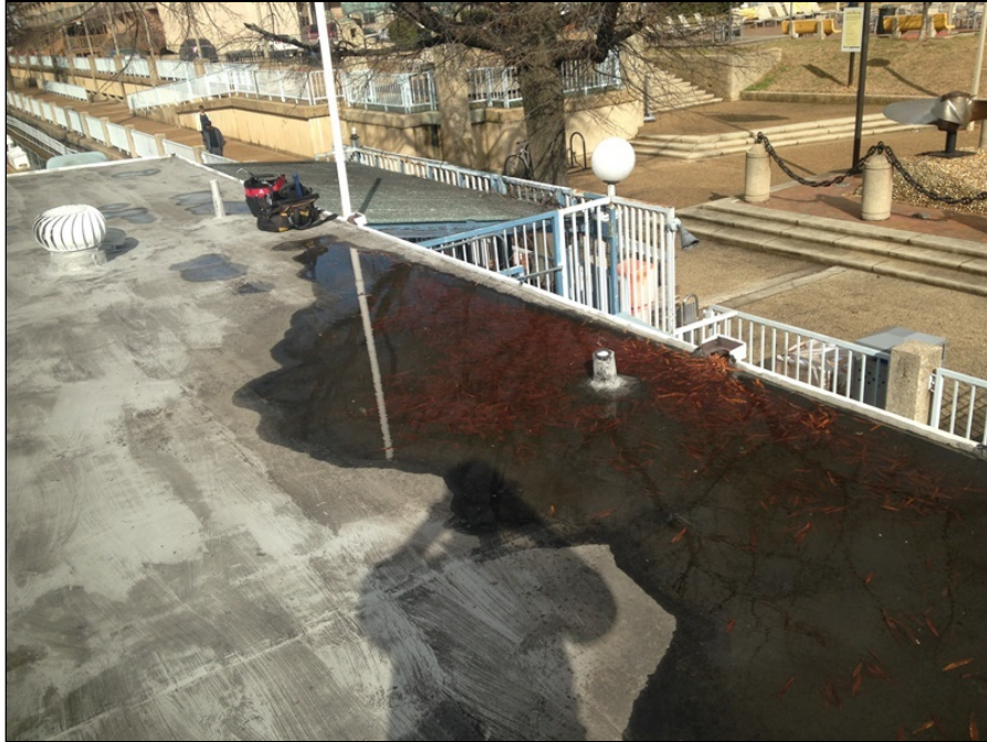
3 - View of the Roof of the Building.
