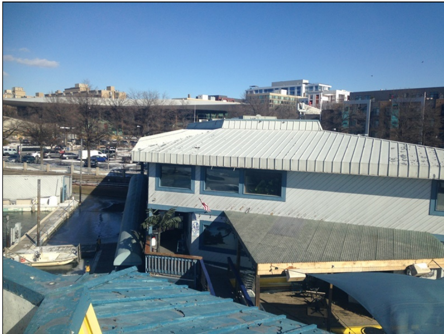
2 - View of Pier 3 Office Building.
