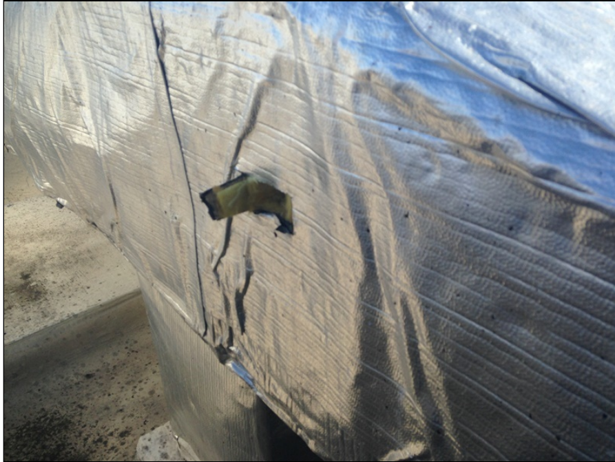
7 - View of Asbestos-Containing Foil HVAC Insulation Wrap on the Roof of the Cantina Marina Building. Sample No. R15.
