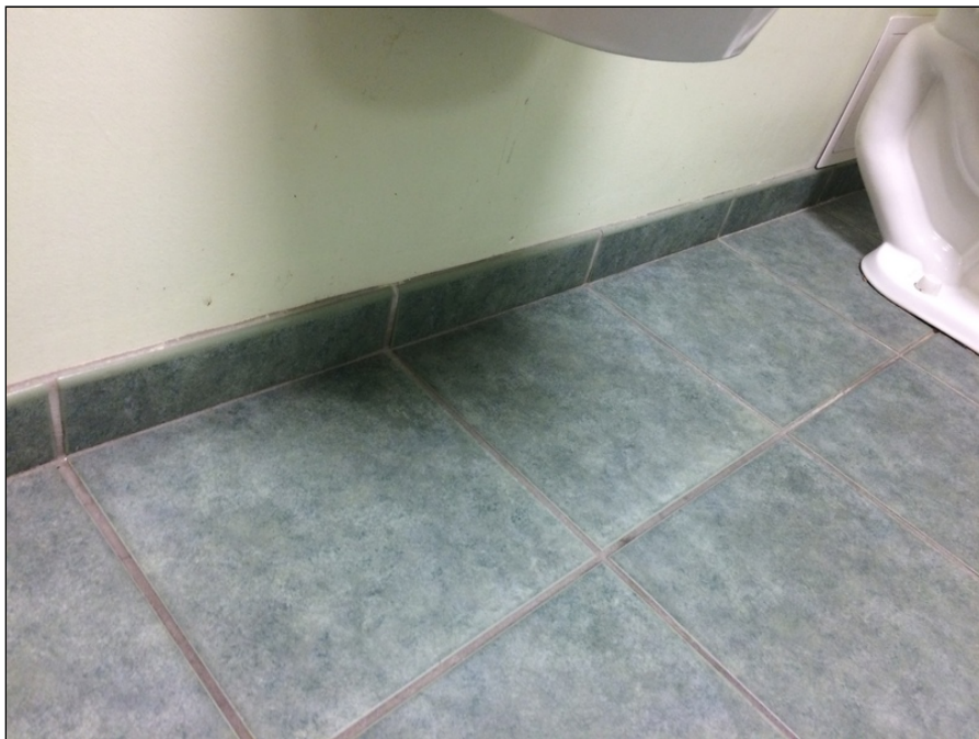
14 - View of Lead-Based Glaze on Green Ceramic Baseboard and Floor Tiles in the Restroom of Cantina Marina. XRF Reading Nos. 87 & 88.
