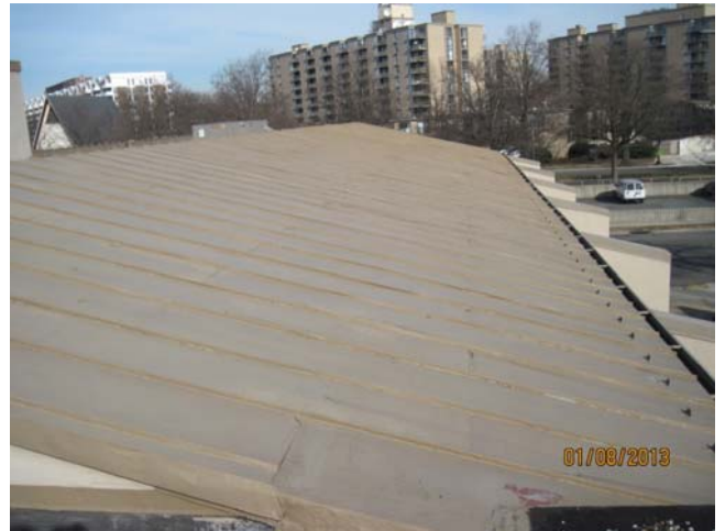
16. View of the assumed brown lead-based paint on the Hotel's tin roof.
