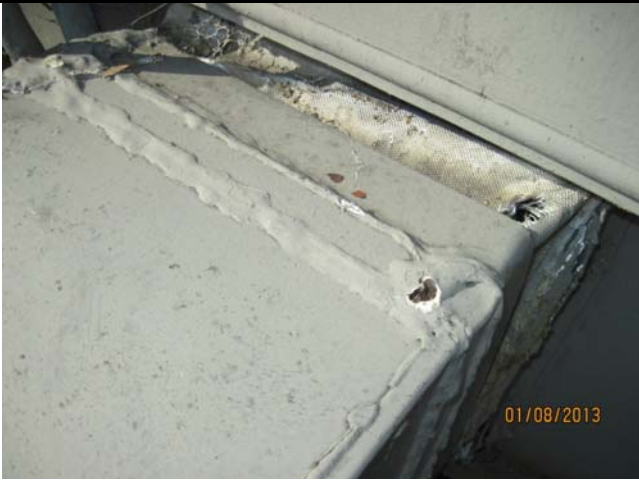
7. View of cream caulk on roof mechanical vent. Samples CI78-CI80
