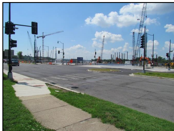
Photo 6: View of the existing signaled intersection installed on Maine Avenue, SW, as part of the Wharf development
